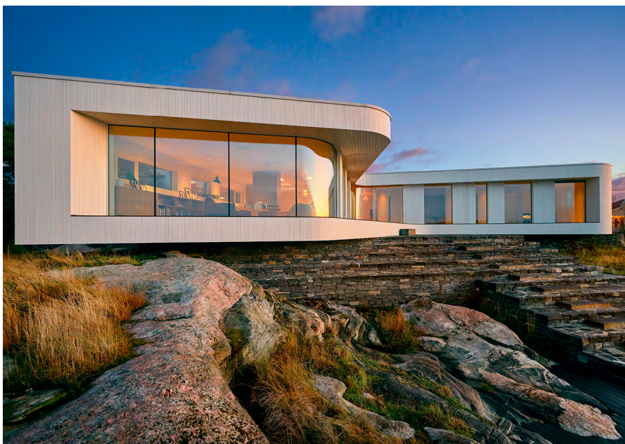
Villa AT | Søgne, Kristiansand, Norway Saunders Architecture (Todd Saunders) © Bent René Synnevåg
